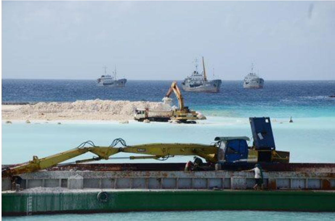
Photo of the construction site at the Sin Cowe Island, which displays the above two approaches to harbor excavation and land reclamation on one of the Spratly Islands by Vietnam
